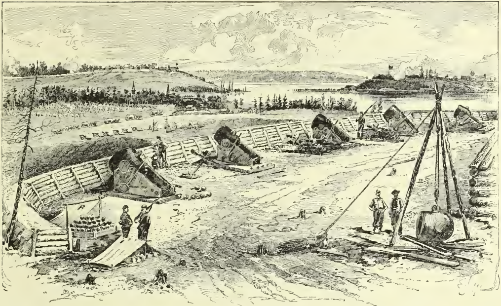
VIEW FROM UNION MORTAR BATTERY NO. 4, LOOKING TOWARD YORKTOWN.—GLOUCESTER POINT ON THE RIGHT. FROM A SKETCH MADE APRIL 16, 1862.
